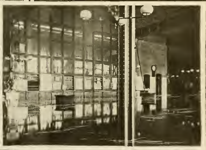
HIGH WATER MARK IN THE BALTIMORE & OHIO STATION AND TUNNEL IN PHILADELPHIA.
